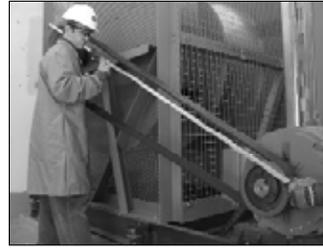
*Using a straight edge to check alignment*
